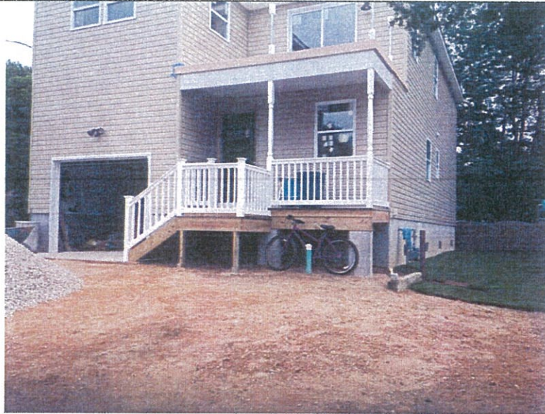
90 Dock Avenue, Front, 7/23/13
