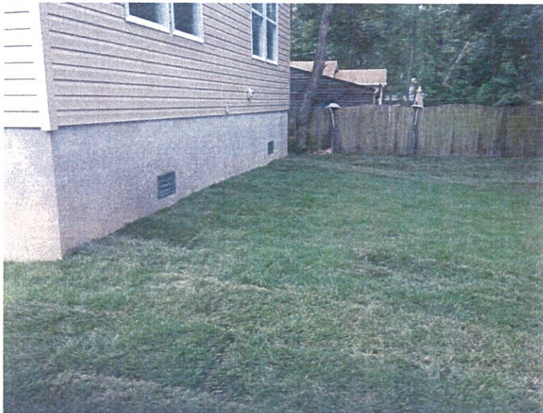
90 Dock Avenue, Rear, 7/23/13
